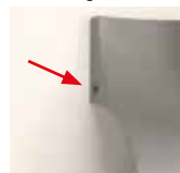
stainless steel dowel for locking the cover
